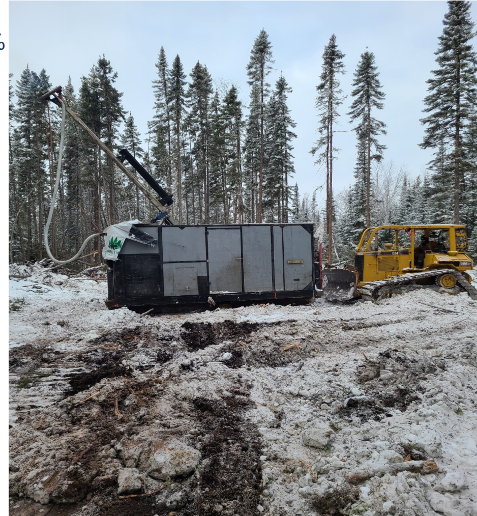
Drilling the Oakes Gold Project in 2022
